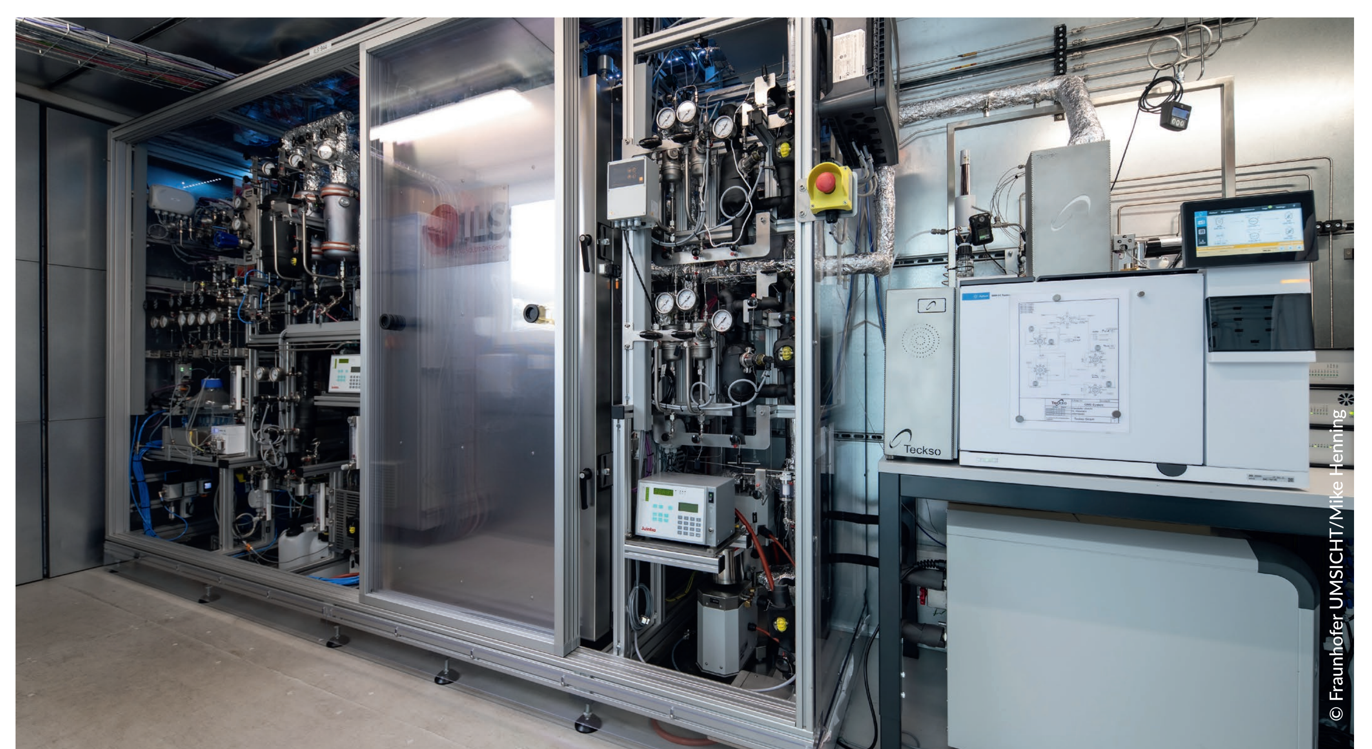
View into the experimental container for thermo-catalytic oxygen removal from steel mill gases in operational environment.
