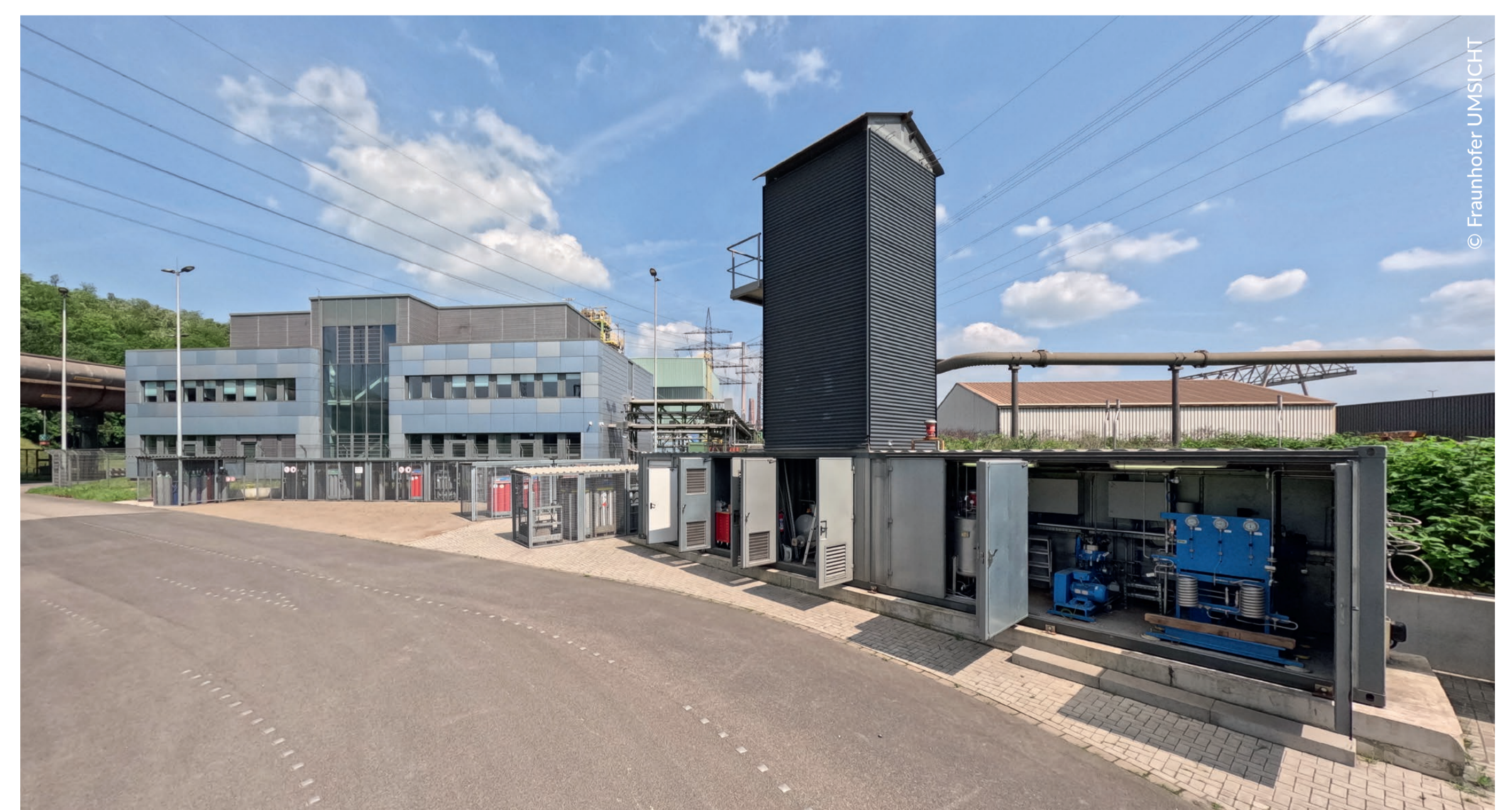
Methanol demonstration plant set-up at Carbon2Chem® technical center.
